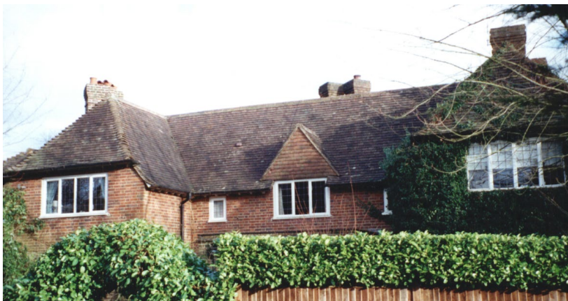
3 & 5 Breech Lane are Arts and crafts style lodges to Little Chesters, a grade II listed building and by the same architects, Nicholls & Hughes of 1927
