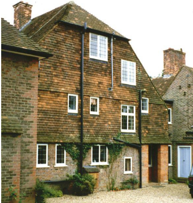
House of 1907 by arts and crafts architect Percy Morley Horder which was remodelled with tile hanging by the notable architect Sir Mervyn McCartney in 1924 for Baron Russell of Killowen family
